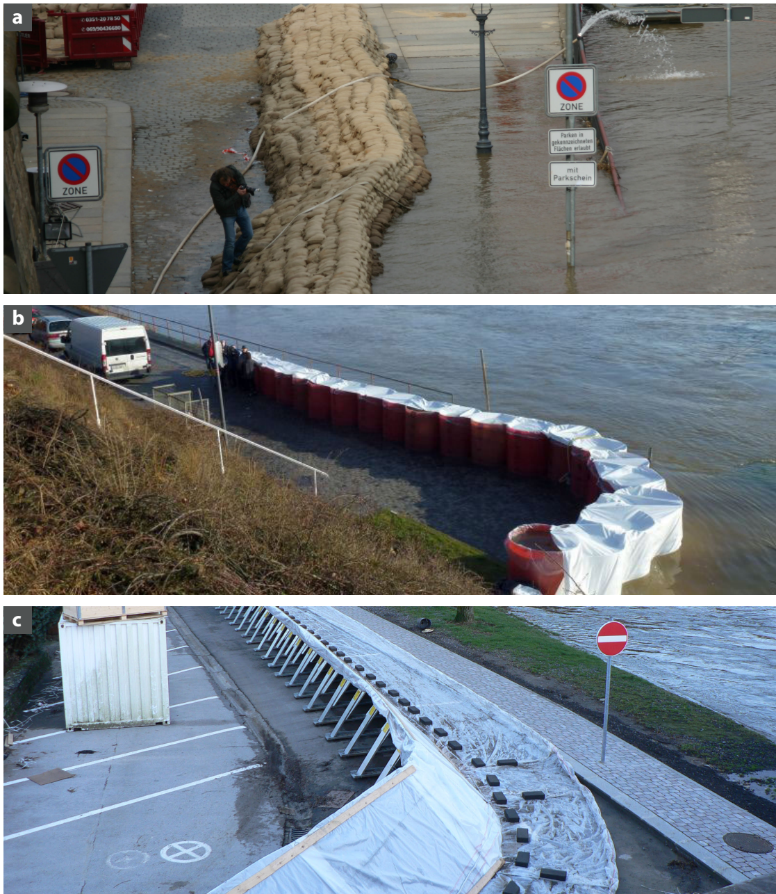
Figure 1.4: Examples of short-term flood protection measures. (a) Sandbags. (b) AquaRiwa. (c) Aquabarrier.
