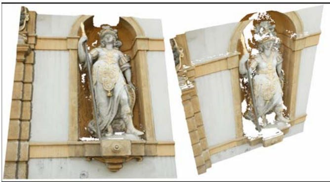
Figure 10. The model with a texture synthesized from all available seventeen input images. Regions which are not visible in any view can not be reconstructed and therefore also have no texture. Examples of such holes are shown in the image on the right hand side.
