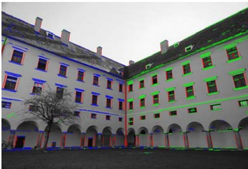
Figure 6. Extracted lines in of the input images. Automatically extracted vanishing points are used to improve and to classify the 2D line segments.
